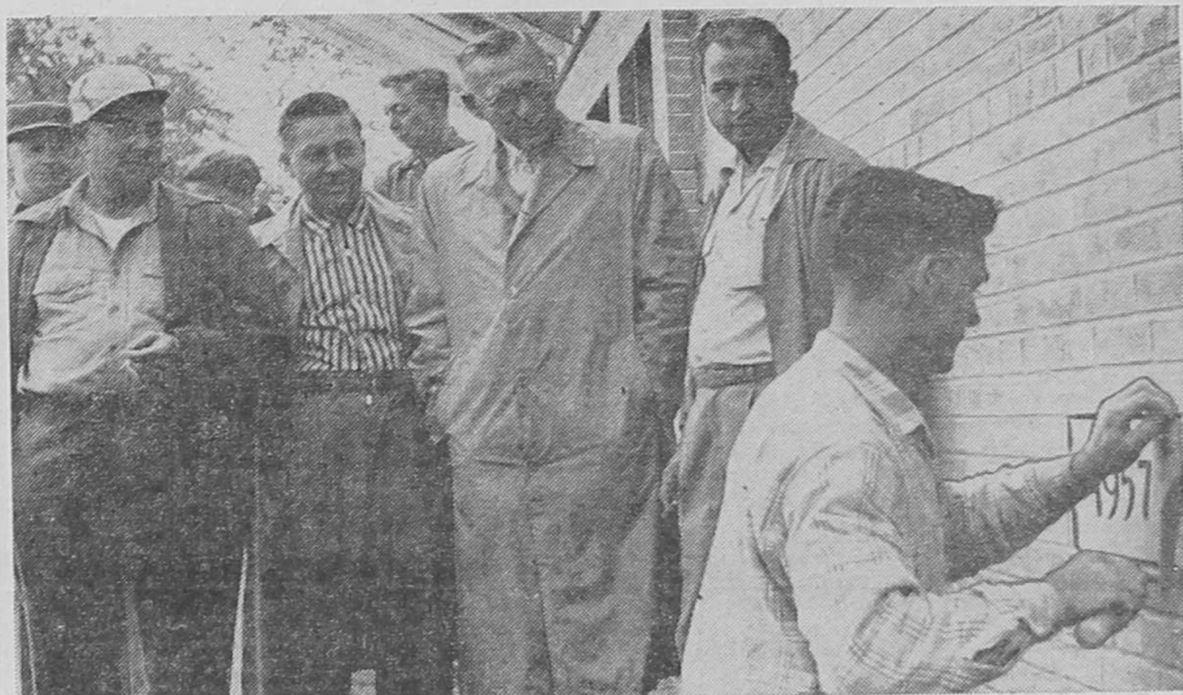
THEY ALSO SERVE who only stand and watch as workman installs cornerstone of Local 291's new $40,000 home in Oshkosh, Wis. From left, C. E. Bergquist, local financial secretary-treasurer; Wesley Doermer, building committee member; Ralph Koenig, Region 10 education and PAC director; Alfred Hoffmann, guide of the local; Region 10 Director Harvey Kitzman, and James L. Reiff, local president.
