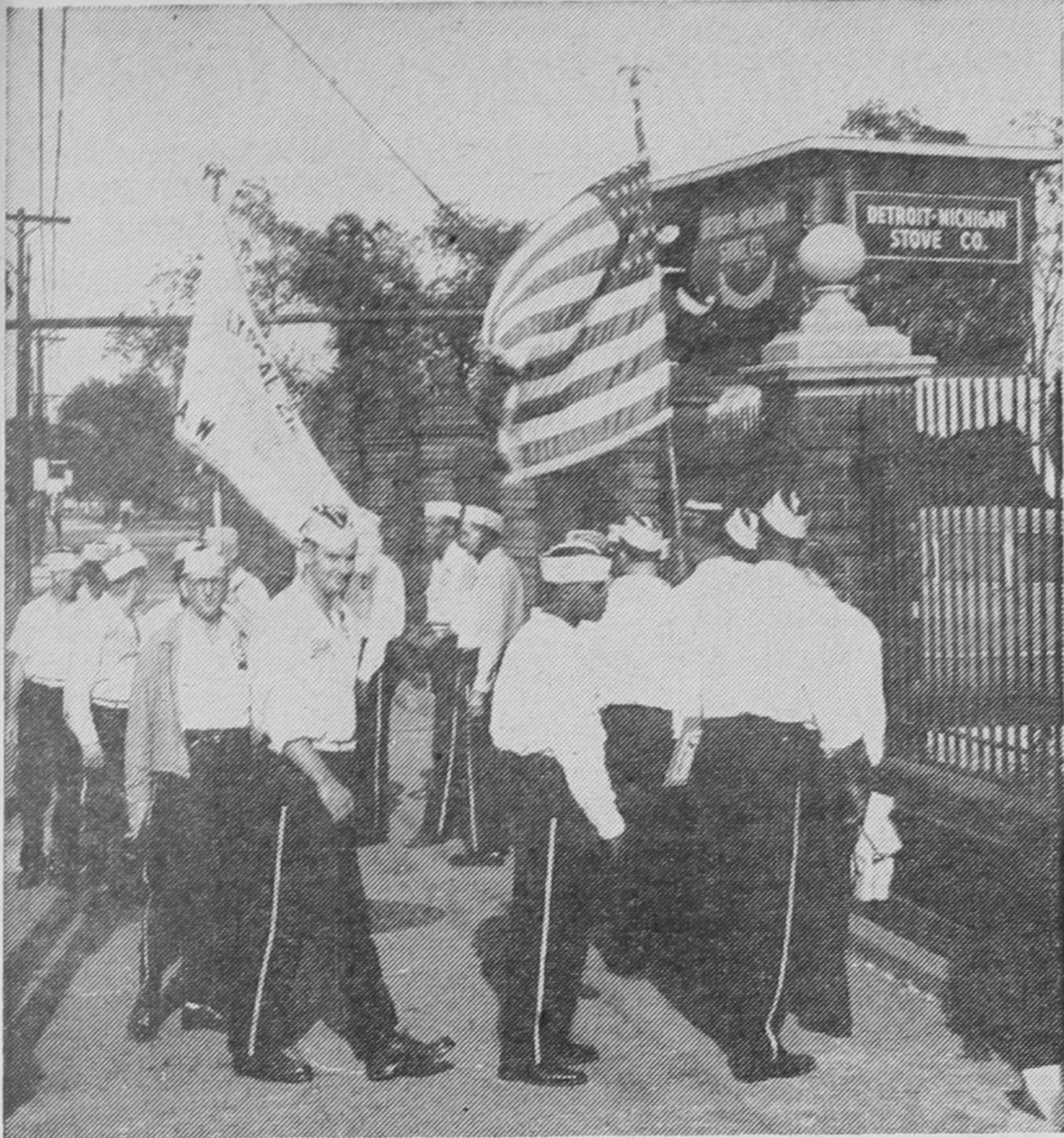
Organization of workers at the Detroit-Michigan Stove Company was aided by workers from other locals in Detroit. Above, members of Briggs Local 212 demonstrate their support of the stove workers in front of the plant.
