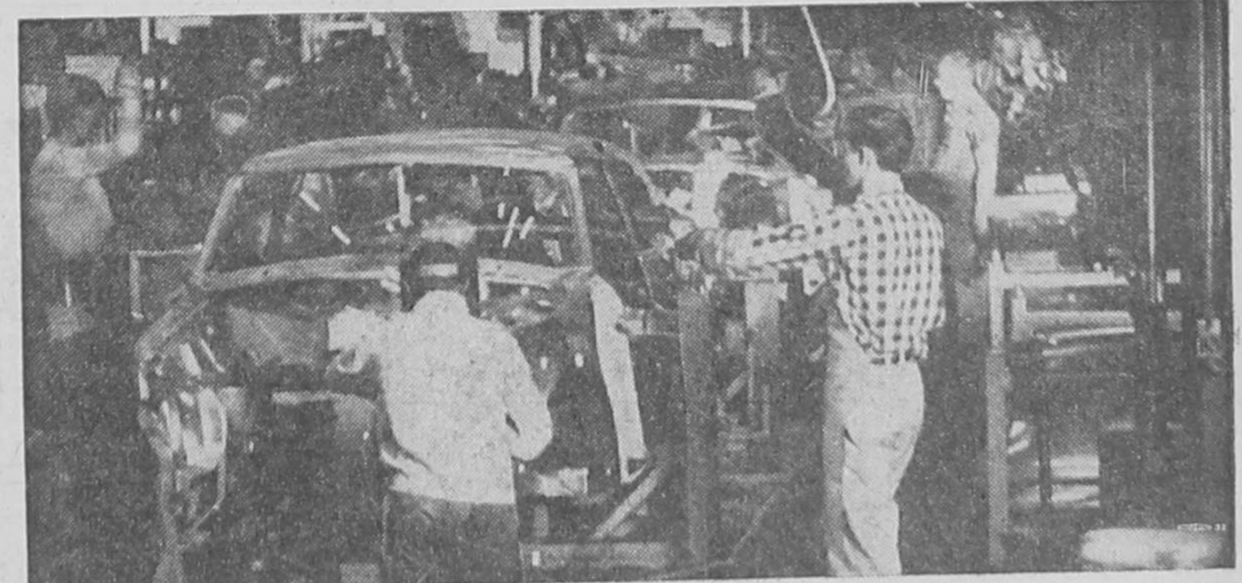
OPERATIONS OF ASSEMBLY LINE are shown in film on Auto Workers' skills as part of AFL-CIO "Americans at Work" television series. Here welders are shown attaching auto body to frame. The AFL-CIO's television program, "Americans at Work," is now being telecast over station WWJ-TV in Detroit, Michigan, at 12:30 p.m. every Sunday.
