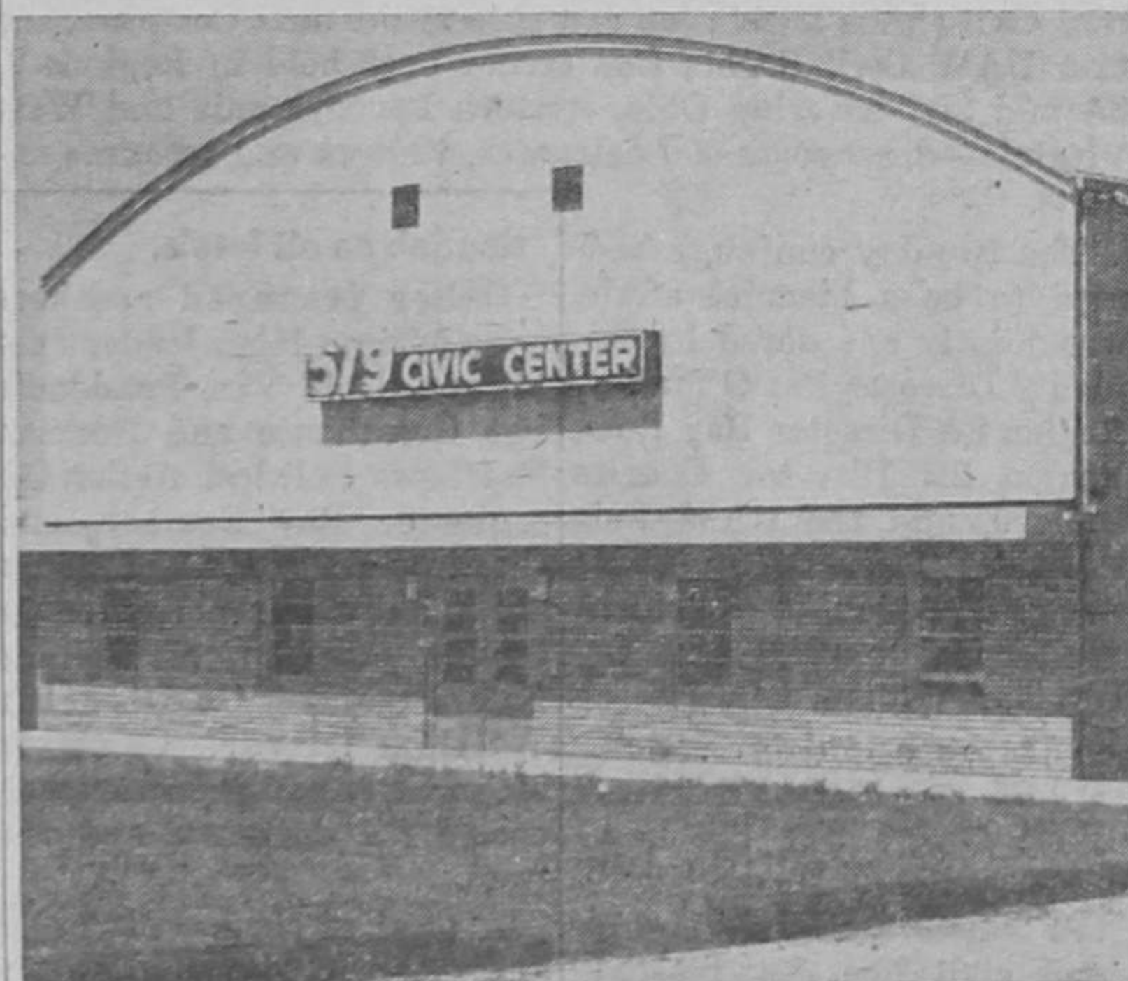
THE MEMBERSHIP is justly proud of Local Union 579's new $100,000 home. The structure, on the outskirts of Danville, Illinois, has an auditorium with a seating capacity of 2,000; a full set of conference, office and recreational facilities.
